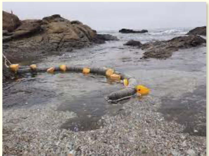
Booms with fiber filled tubes soaking up oil
